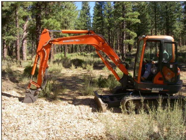
FIGURE 5. KX 161 EXCAVATOR TARGETED LOOSENING.
