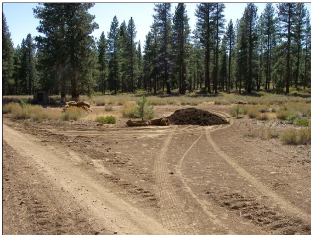
Figure 3. Ripping with the modified excavator bucket on plot 1.
