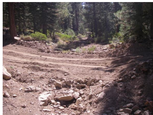
Figure 7. Haul road crossing ephemeral drainage near Dry Lake (hot spot 3). Filled in crossing is a potential source of sediment.
