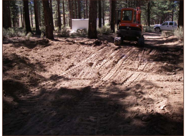
Figure 4. Track packing rolling dip. Basin is on the left (PPC).
