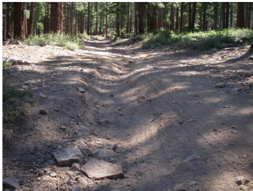
Figure 2. Water capture and gully formation on Sawmill Road.
