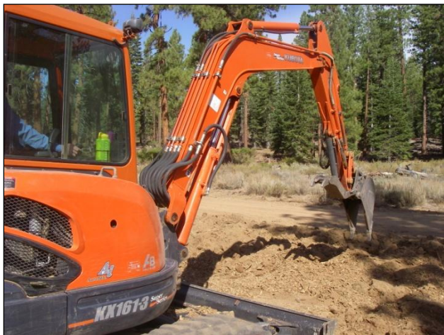
Figure 3. An example of ripping with a modified excavator bucket.
