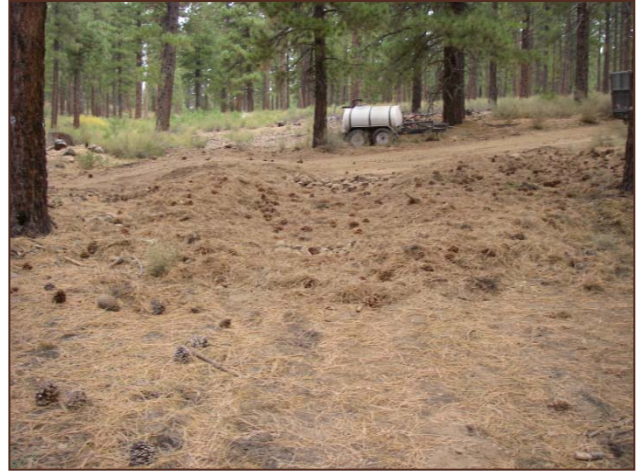
Figure 8. Site post construction (PPB).
