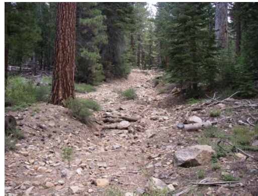
Figure 3. Used as a haul road in 1994-95, the entire road bed has since been eroded down to rock due to capture and concentration of surface runoff. In 2009, this road was allowed to be regraded for use as a haul road once again.
