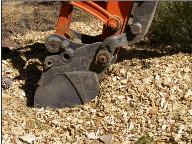
FIGURE 3. MODIFIED EXCAVATOR BUCKET AT FULL PENETRATION.
