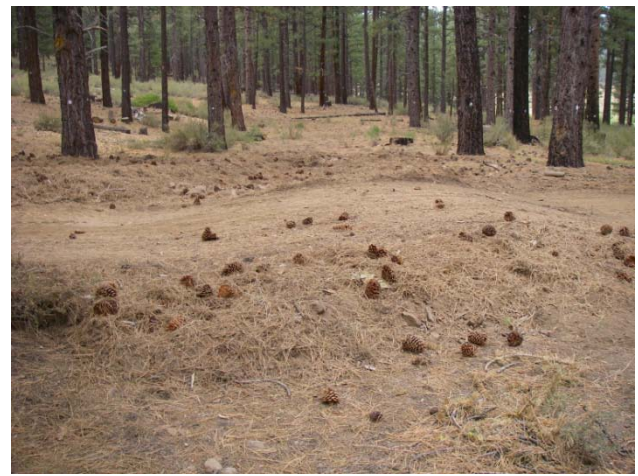
Figure 4. Track packing rolling dip. Basin is on the left (PPC).
