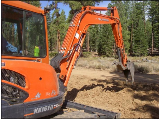
Figure 3. Ripping with a modified excavator bucket.
