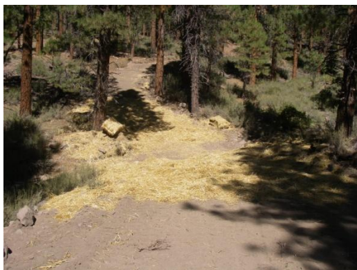
Figure 6. Haul road crossing ephemeral drainage (hot spot 6). Straw was spread on the road surface at the crossing as a BMP.
