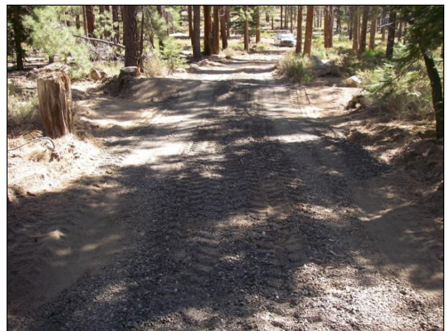
Figure 6. Compacted asphalt grindings on plot 2E
